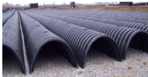
Figure 1-6. Subsurface infiltration system, generic example (Source: Conteches.com)
