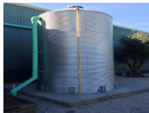
Figure 1-8. Rainwater harvesting cistern, Environmental Innovation Center, San José (Source: City of San Jose)
